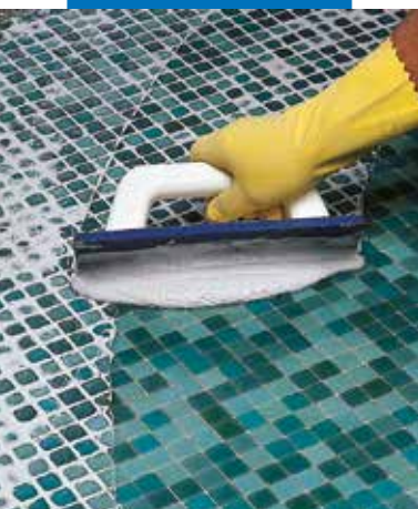
Grouting glass mosaic with Keracolor FF mixed with Fugolastic
